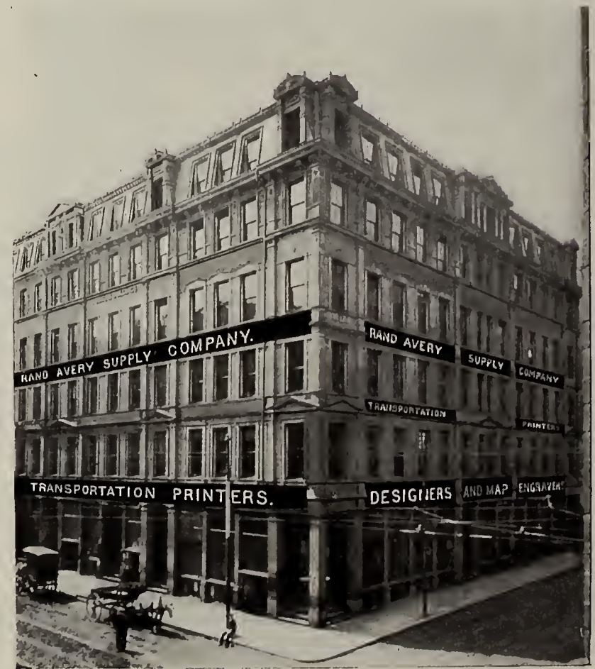
RAND AVERY SUPPLY CO.'S BUILDING, 117 to 123 Franklin, and 61 to 71 Federal Streets, Boston.
